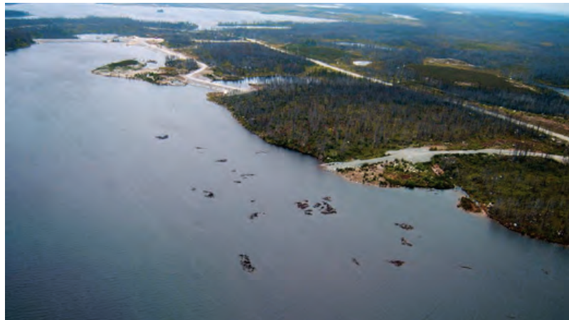
Floating peat islands near the boat ramp upstream of Lemare dam.
