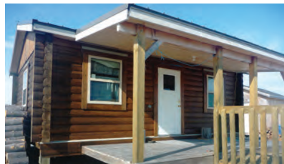
After the maintenance and restoration
